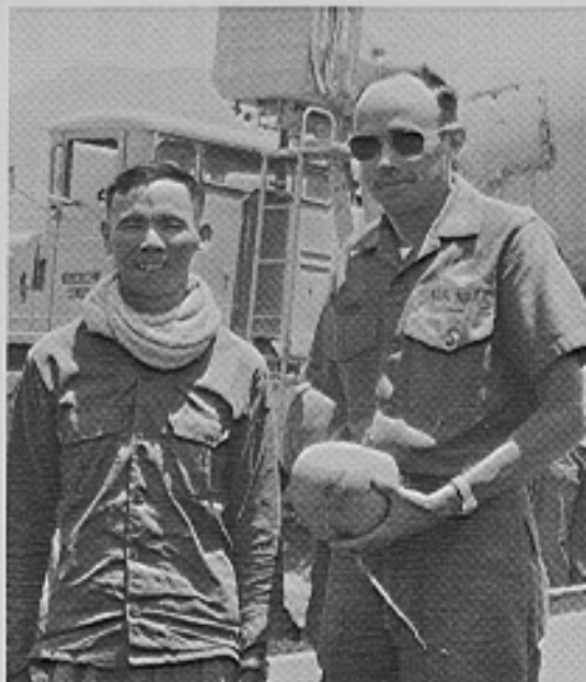
Village leader (left) and Lcdr P.R. Winn watch construction in progress
